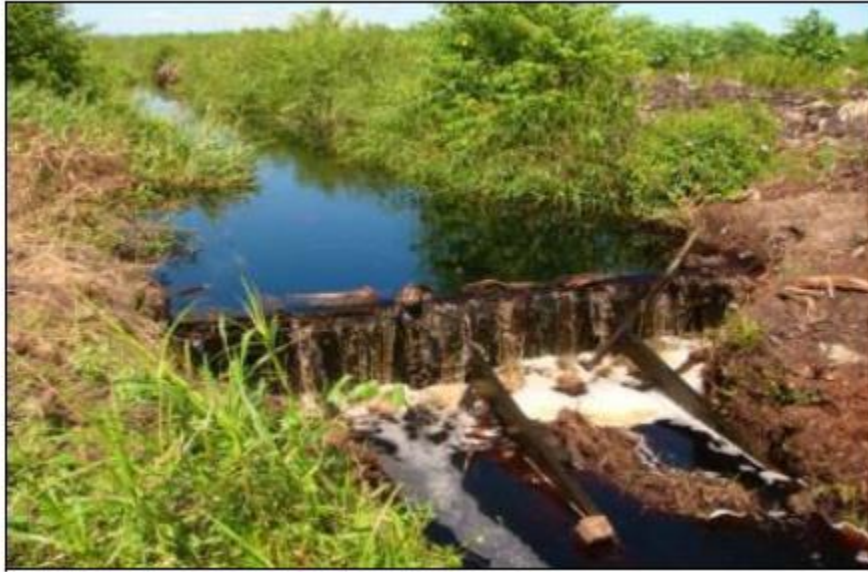
Timber Log Check Dam
