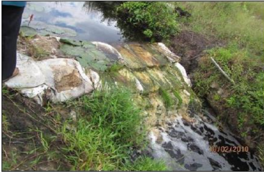
Typical Sand-Fill Bag Check Dam
