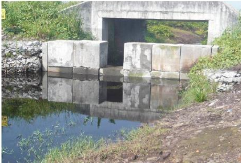
Precast Concrete Block-Section Check Dam
